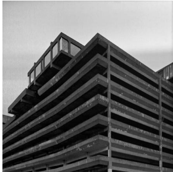
Trinity Square Car Park, Gateshead, 1962-1967. Architect: Rodney Gordon for the Owen Luder Partnership
